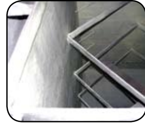
After: Completed application silo surface restored
