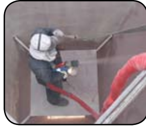
Application of Defend-X® by certified technician
